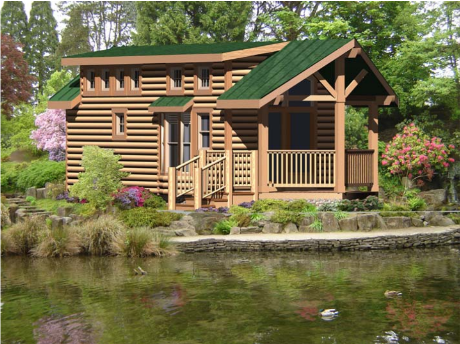
Artists conceptual rendering featuring optional covered porch, log siding, and metal roof.
